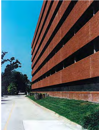
Parking Garage: Auto-Oriented Façade
