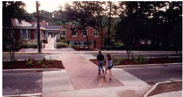
A traffic-calming measure that improves the pedestrian environment by slowing traffic. Source: (11).
