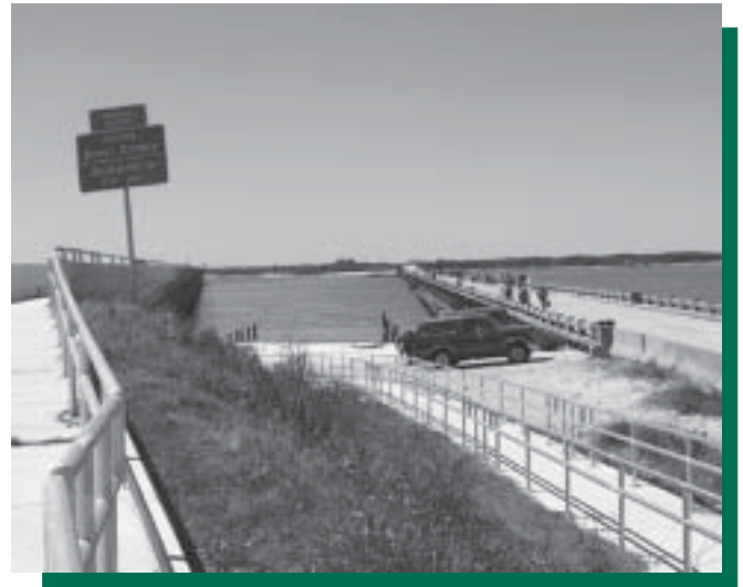
Nassau Sound Bridge
