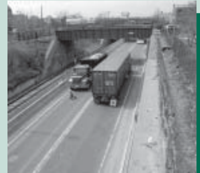
South Boston Haul Road
